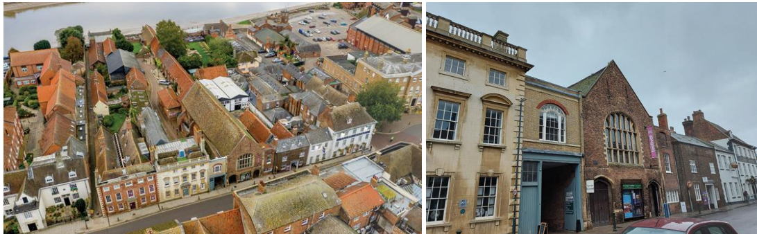
Figure 8 – Aerial and Front View of the Guildhall
